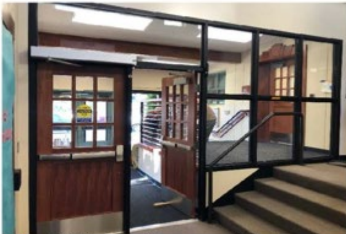
Central ES: A view of the new vestibule from the interior of the school.
