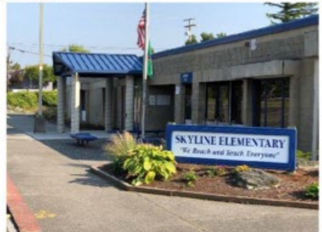
Skyline ES: A view of the new entry canopy at the secured vestibule entrance.
