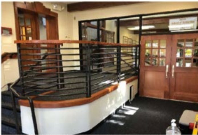
Central ES: The new entry vestibule is now complete.
