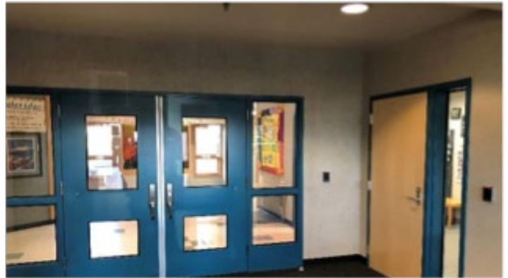
The Eagleridge secured entry & vestibule has been completed. It includes video buzz in entry. The secure entry forces all visitors to go through the office before being allowed access into the school.
