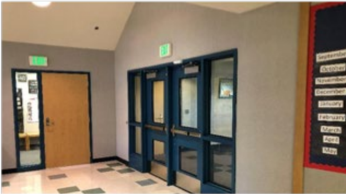
This interior photo at Eagleridge shows the new wall framing and relocated secondary door system.
