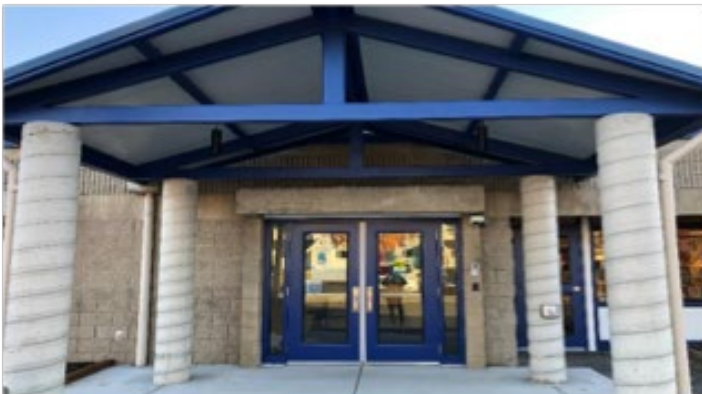
The new Skyline secured entry is also complete. There is now a clear designated entry for visitors with the same enhanced security features.
