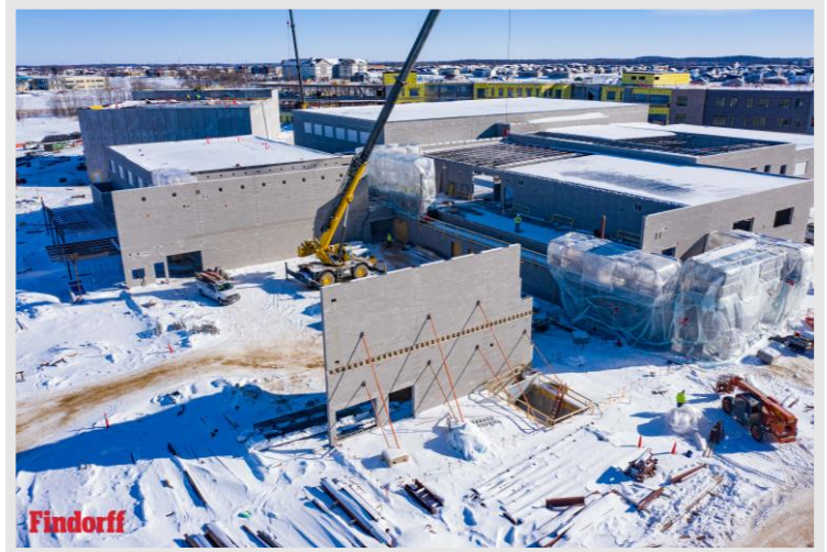
Masons are building block walls adjacent to the Pool. Steel roof joists and decking will follow.
