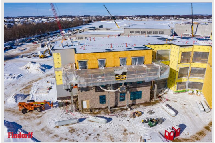
Brick façade is being installed by the masonry crew on the south side of the Learning Communities.
