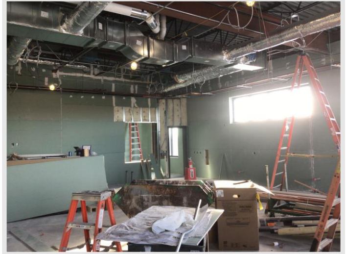
Drywall is well underway in the Learning Communities, giving the rooms their true enclosed shape!
