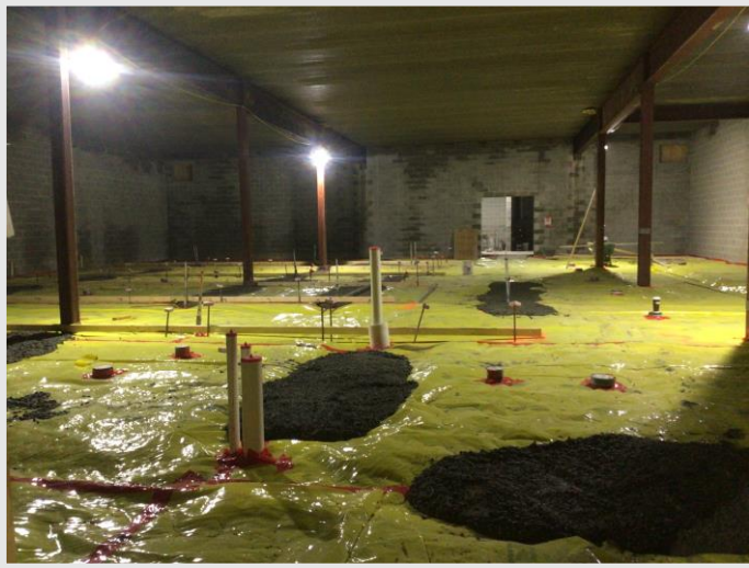
Concrete slab on grade at the Locker Rooms is underway, as the first yards of concrete are poured as seen above
