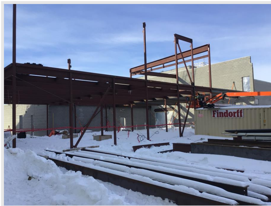
Ironworkers have been setting structural steel in the Teaching Kitchen and Health areas, erecting the second level columns in the last week.
