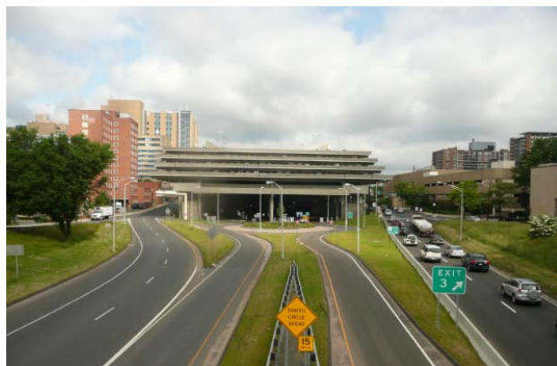
Figure 4.12 – Parking deck – New Haven,
