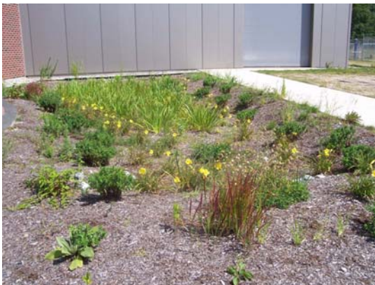
Bioretention area at University of Connecticut Storrs Campus.
