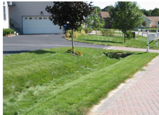
Figures 4.20 – Vegetated drainage way. Photograph courtesy of the University of Connecticut NEMO program, Kara Bonsack
