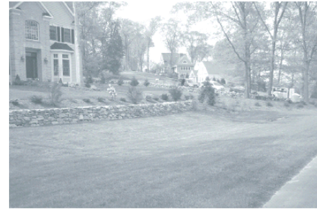
Figure 4.18 – Vegetative filter strip. Source: Connecticut, 2004.
