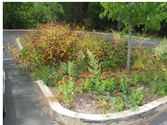
Figure 4.13 – Bioretention in use as a parking lot island in Branford, CT. Source: Connecticut Department of Environmental Protection.
