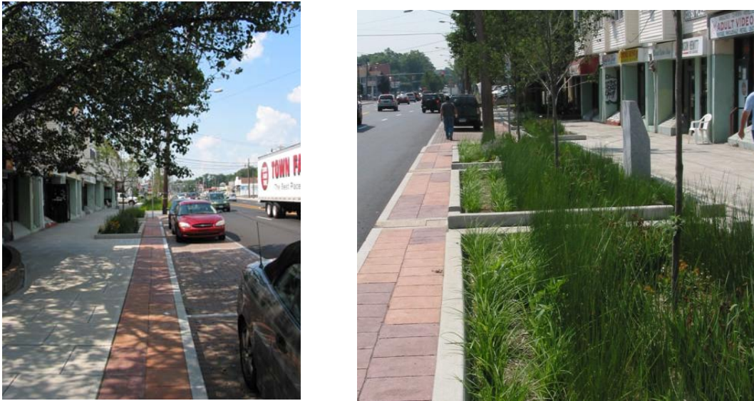
Figure 3.12 – Permeable pavement (left photograph) and rain garden/bioretention (right photograph) retrofits along North Main Street in Bridgeport, CT.
