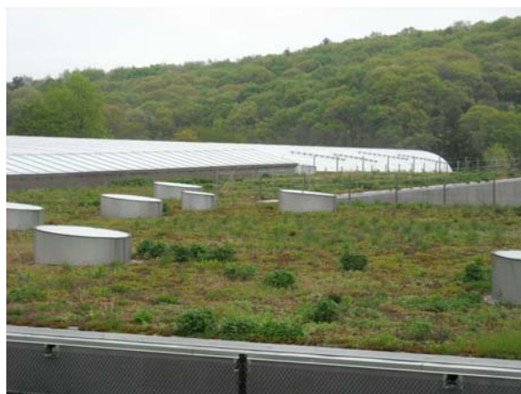
Figure 3.16 – Retrofit and redevelopment techniques in Connecticut. Source: Connecticut Department of Environmental Protection.
