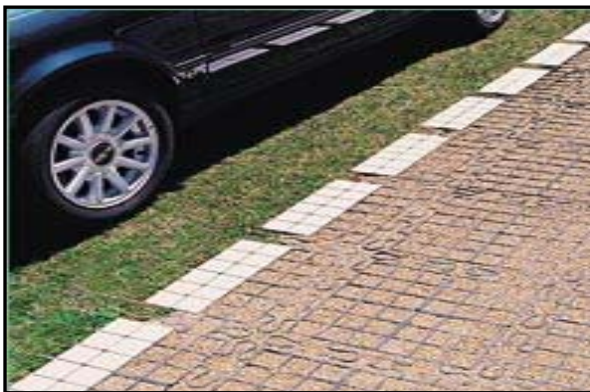
Figure 4.15 – Permeable pavement. Source: Connecticut, 2004.
