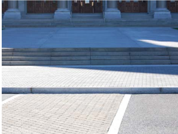
Figure 3.15 – Permeable pavement at Hartford Green Capitols Project. Source: Camp Dresser & McKee.
