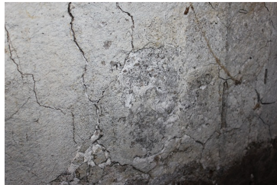
(c) map cracking
