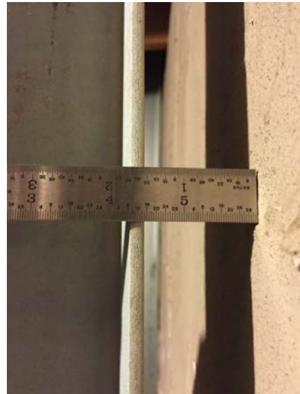
e) significant deformation of the concrete foundation wall
