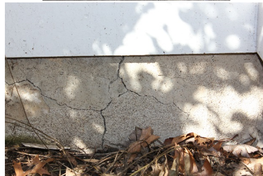
(b) map cracking
