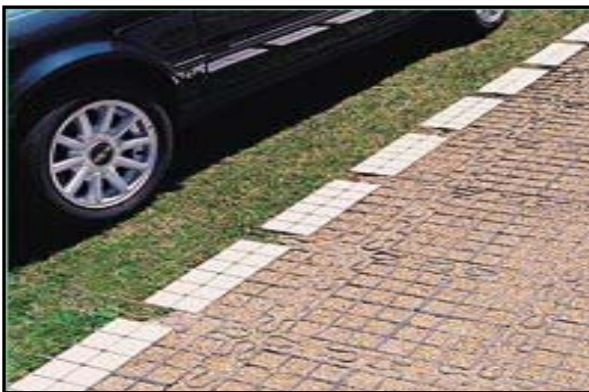
Figure 4.15 – Permeable pavement. Source: Connecticut, 2004.
