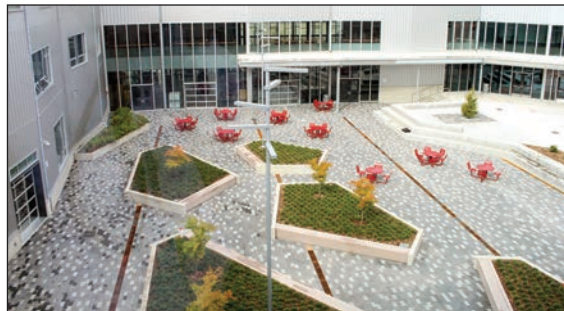
The three-story Juanita High School is built around a center courtyard with outdoor seating and gathering options.
