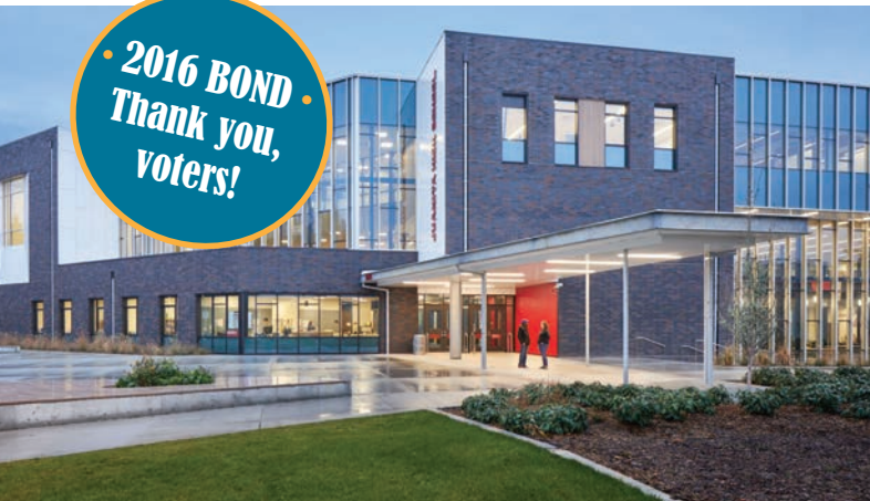
The welcoming entry to Juanita High School. By utilizing GC/CM contracting, the district was able to work with a contractor and our Design and Construction Advisory Committee early in the design process to create a plan that allowed construction to be completed one year early.
