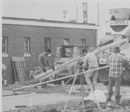
Above: Cafe expansion getting underway in April '96.
