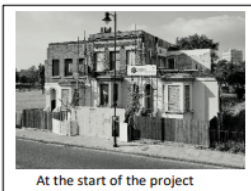
At the start of the project
