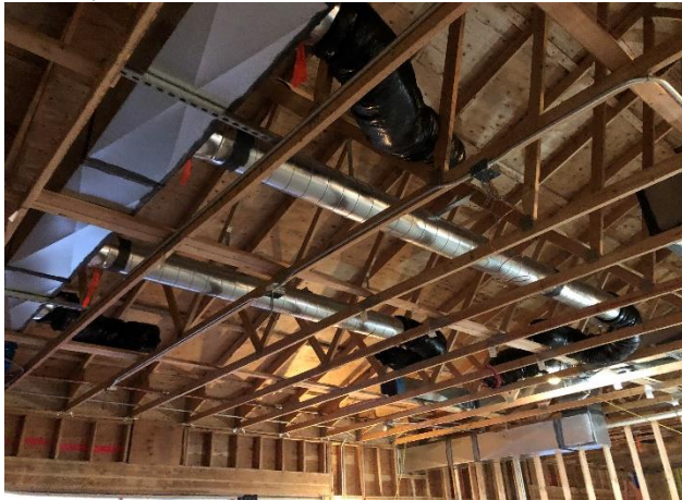
Ductwork is proceeding overhead in the classrooms.
