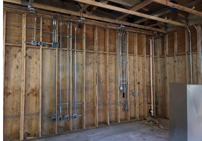
Electrical conduits are being installed throughout the new classroom addition.
