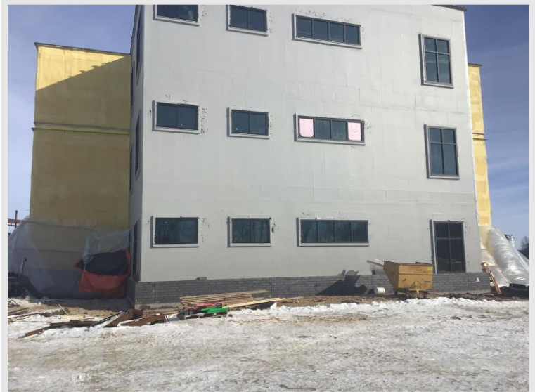
Masons have begun installing the brick façade (dark brick, bottom of the wall) on the far west side of the Learning Communities.
