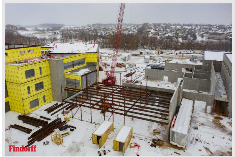
Ironworkers erecting steel columns and beams in the Loading Dock / Kitchen area.
