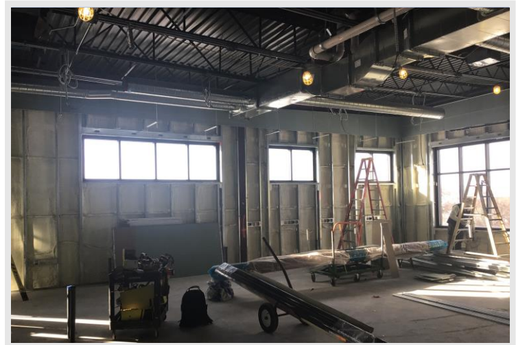
Above ceiling rough-ins are underway, along with insulation and framing at the 3 rd Floor of the Learning Communities
