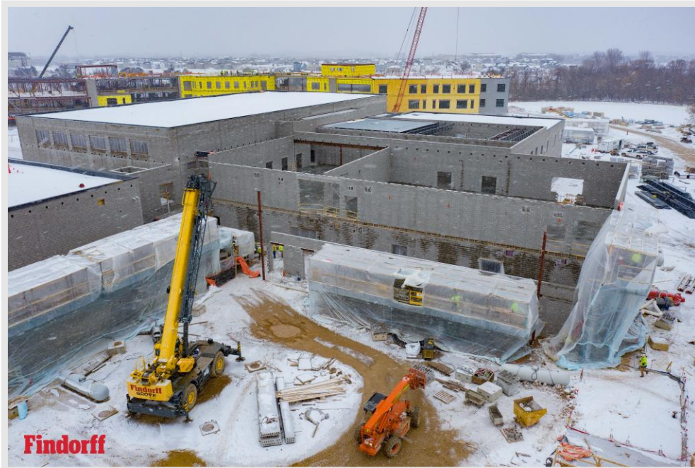
Masons are installing block walls in the Pool and lobby west of the Auxiliary Gym.
