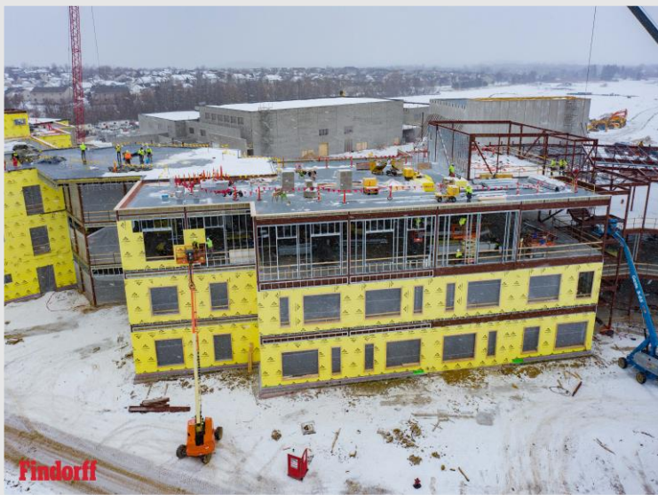
Carpenters installing exterior steel stud walls and sheathing on the southern-facing walls of the Learning Communities.
