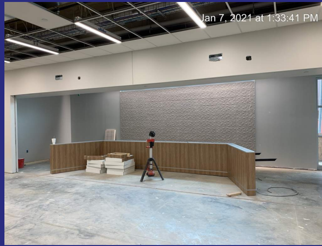
Board Room - Paint, Tile, Casework
