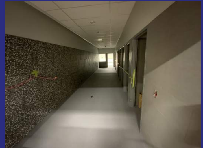
Epoxy Floor - Area B LVL 1
