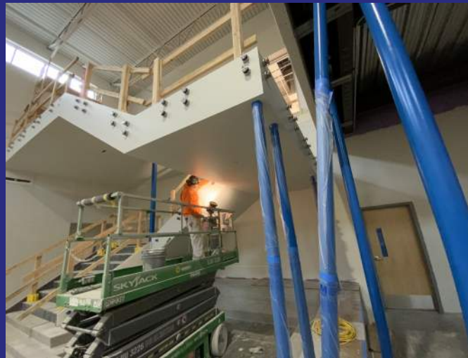
Media Stairs - Paint
