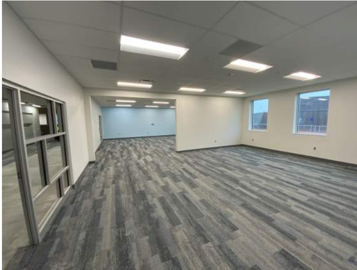
Finishes - Area B LVL 1
