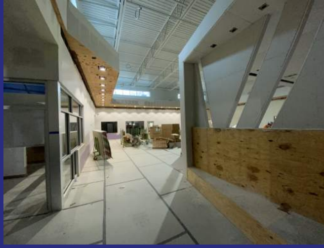
Common Area - Rough In & Drywall
