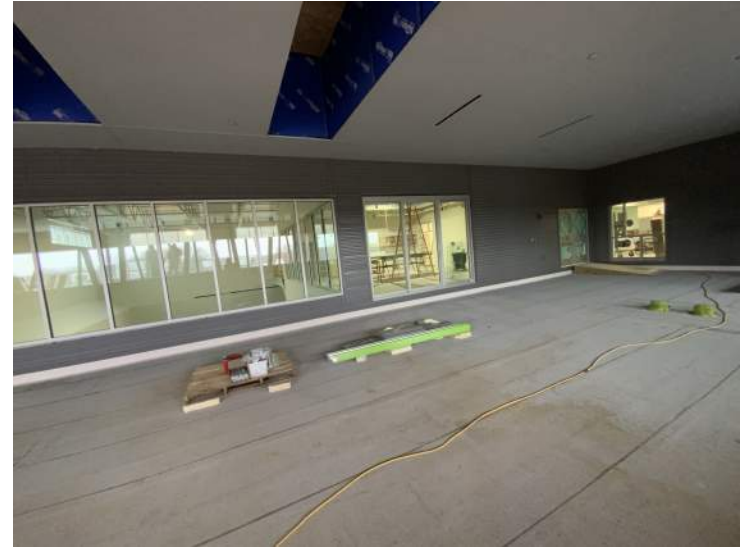
Outdoor Classroom - Siding
