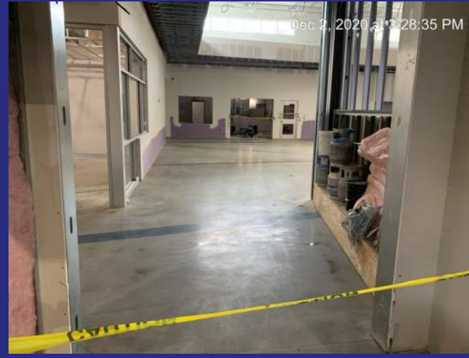
Area A - Floor Polish Underway
