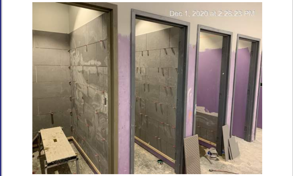
Area B LVL 2 - Tile Install
