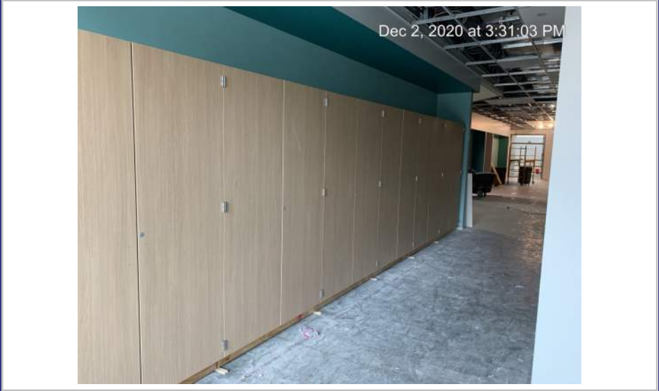
Area B LVL 2 - Paint and Cabinets
