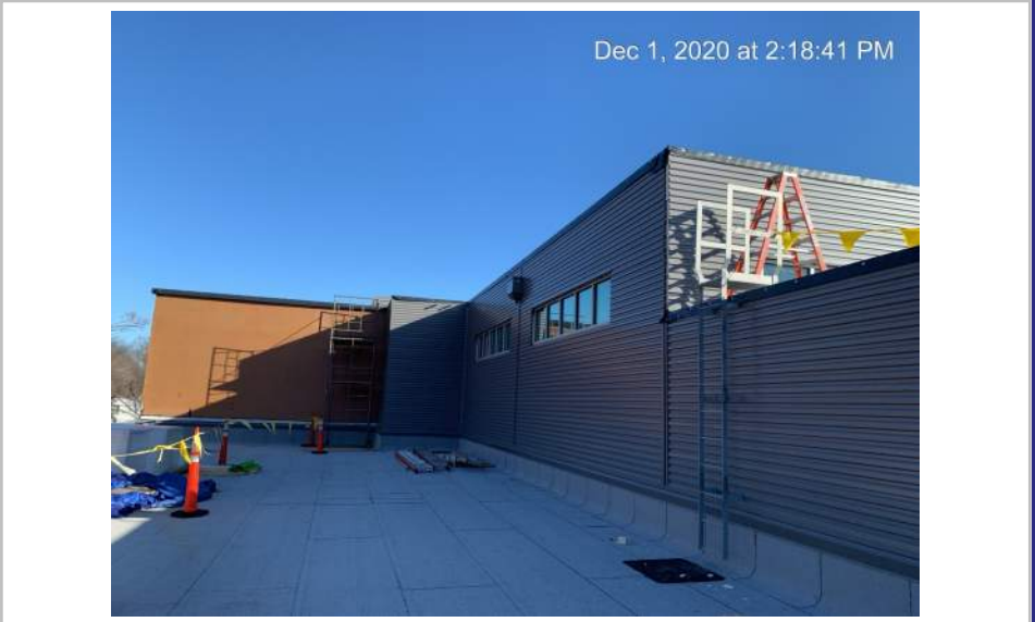
North Building - HR-16 Panel Siding Installation
