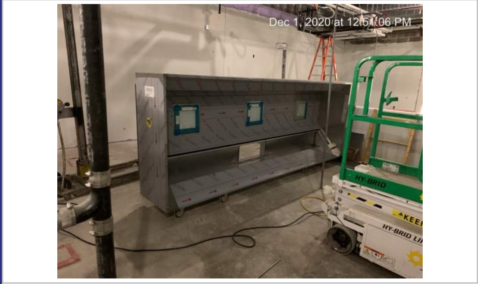
Kitchen Hood Install
