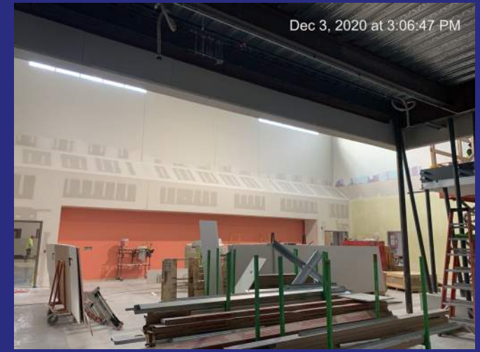
Area A - Drywall
