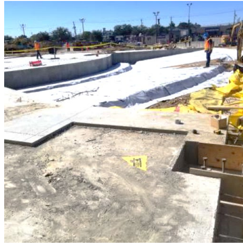
Prepping lower seating area of Auditorium for concrete pour
