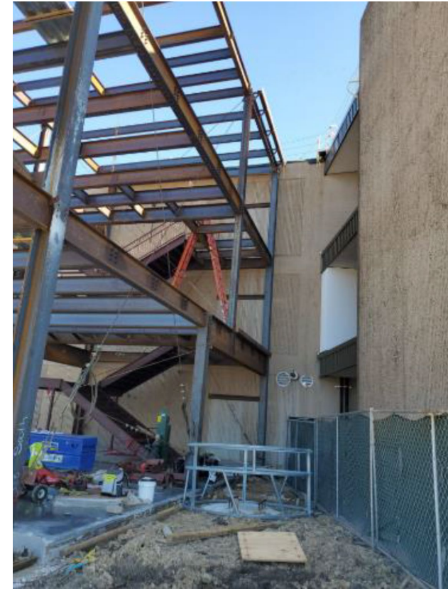
Steel frame next to the existing North stair tower
