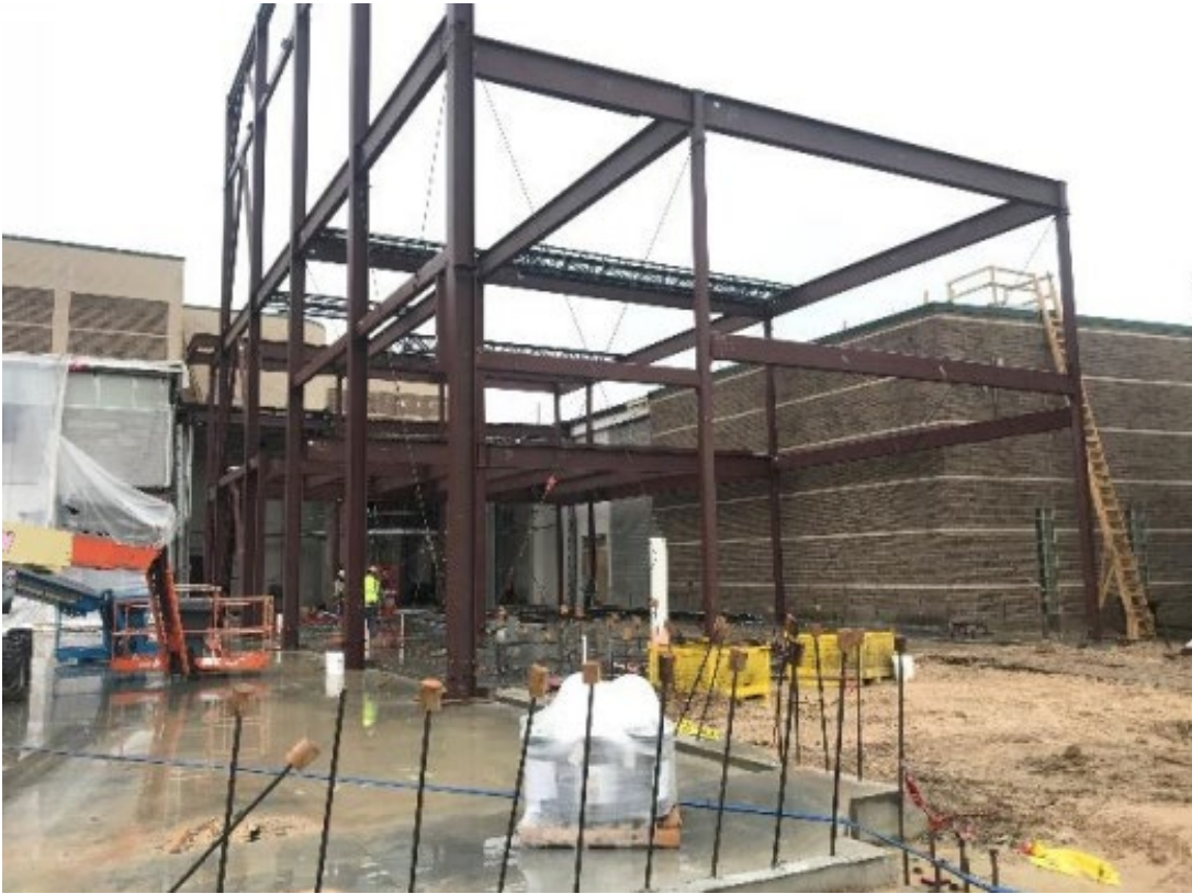
Steel beams and columns are being erected
