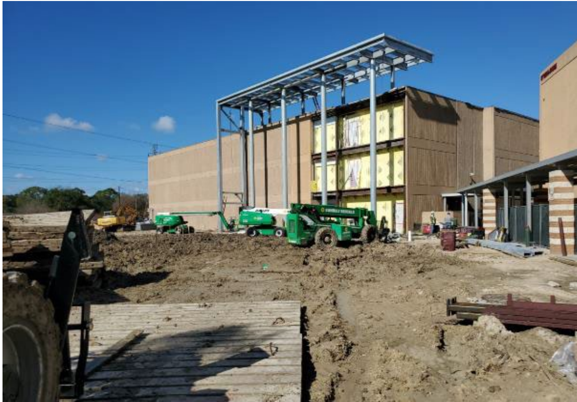
Structural frame for new main canopy has been erected
