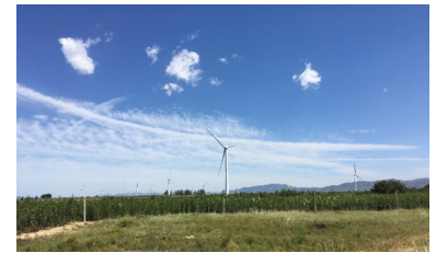
Guanting wind turbine
