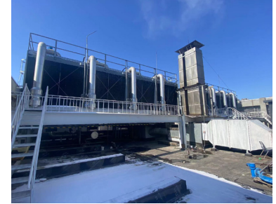
Cooling towers at ISB
