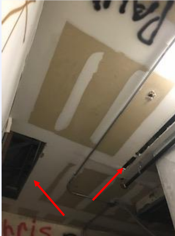
Ducts falling out of ceiling by the access to the house lights
