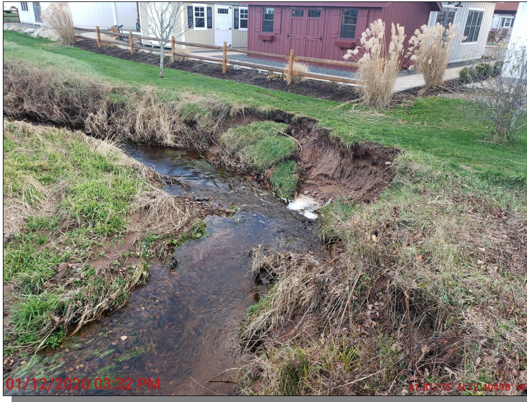
Photo 9: Bank erosion at first bend downstream of culverts; December 2020; facing southeasterly
