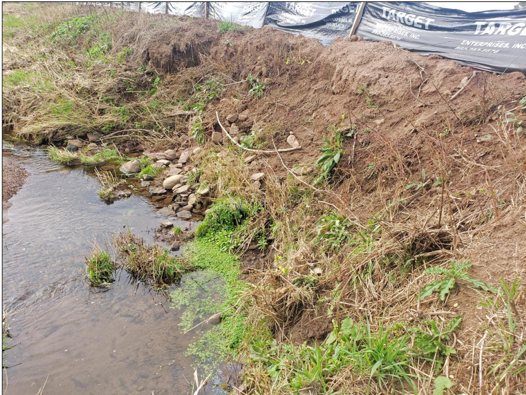
Photo 4: Eroding bank (northerly) at second bend downstream of culverts; facing northwesterly
