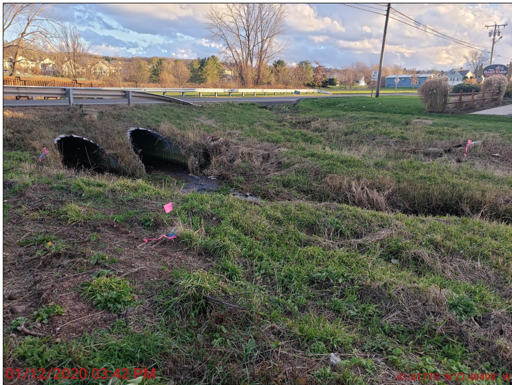
Photo 10: Twin corrugated metal pipes; facing southeasterly
