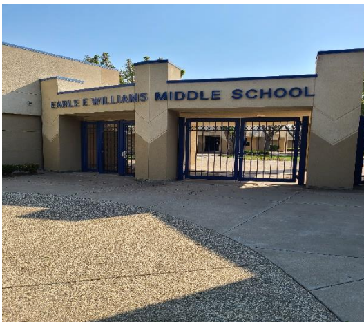
Picture 6: Main Office Gate
