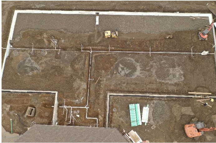
Under slab plumbing was completed, inspected and tested last week.
