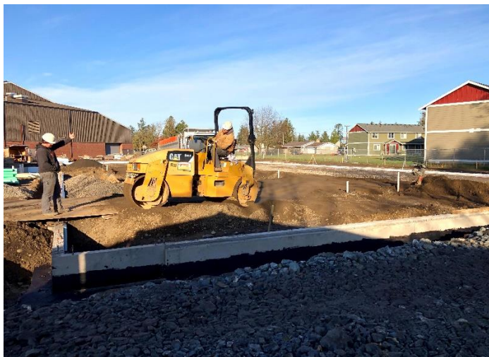
Compaction are underway within the classroom area.
