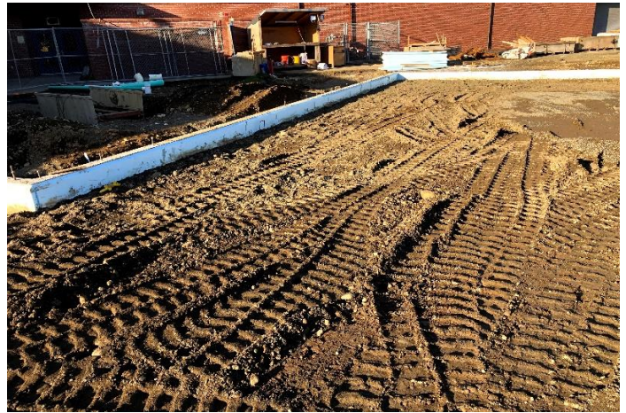
Backfill placement and grading is progressing.
