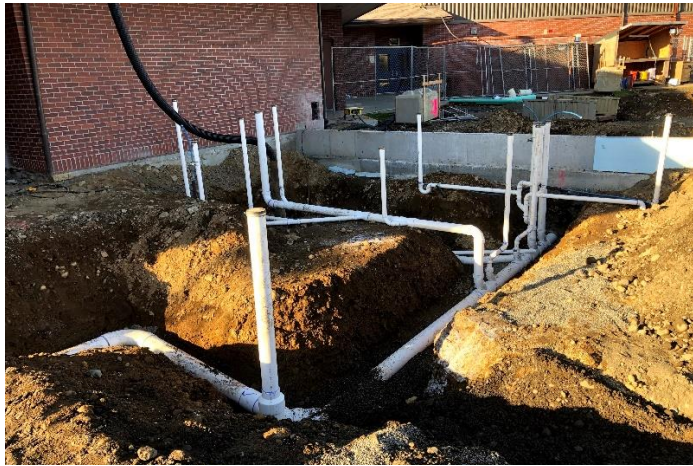
A close up view of the plumbing under the main bathrooms.
