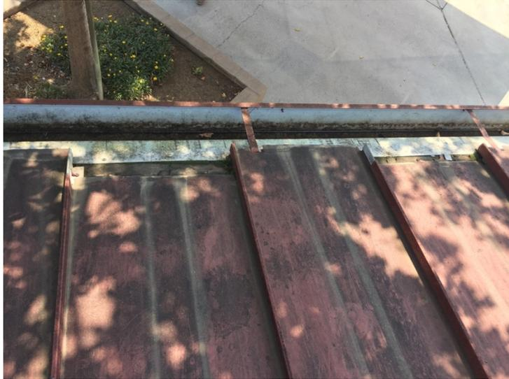
3. The panels are buckling at the ridge resulting in damage to the zee closure and ridge cap.
