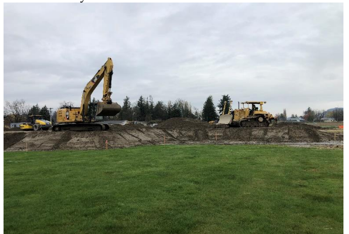
Pre-load and building pad perimeter grading on the east end.
