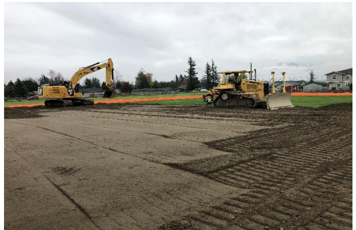
Grading & compaction on the east side of the pad is underway.
