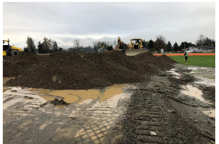
Gravel continues to be brought in, graded and compacted.
