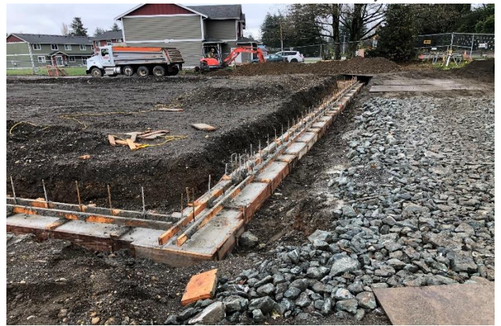
The final section of concrete footings has now been poured.
