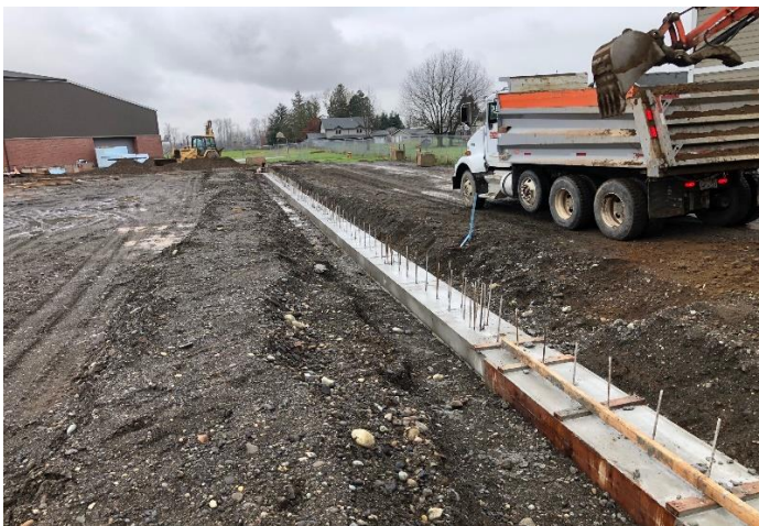
Form removal is underway.
