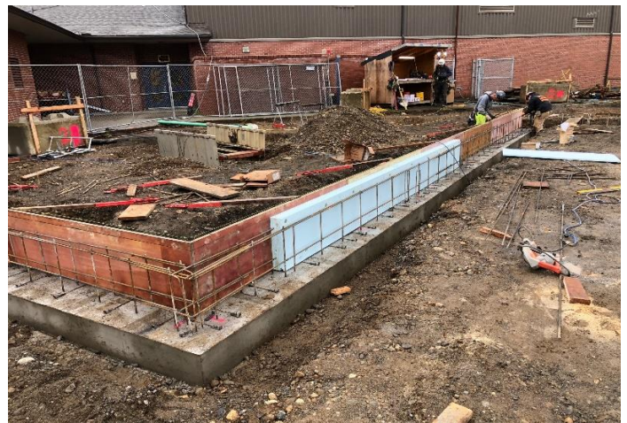
Concrete stem wall forming has now started.
