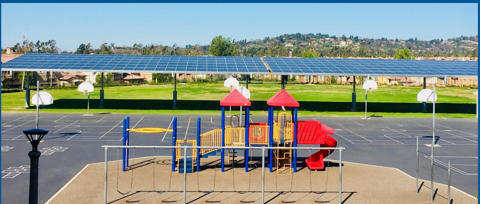
Example of an Elevated Structure
