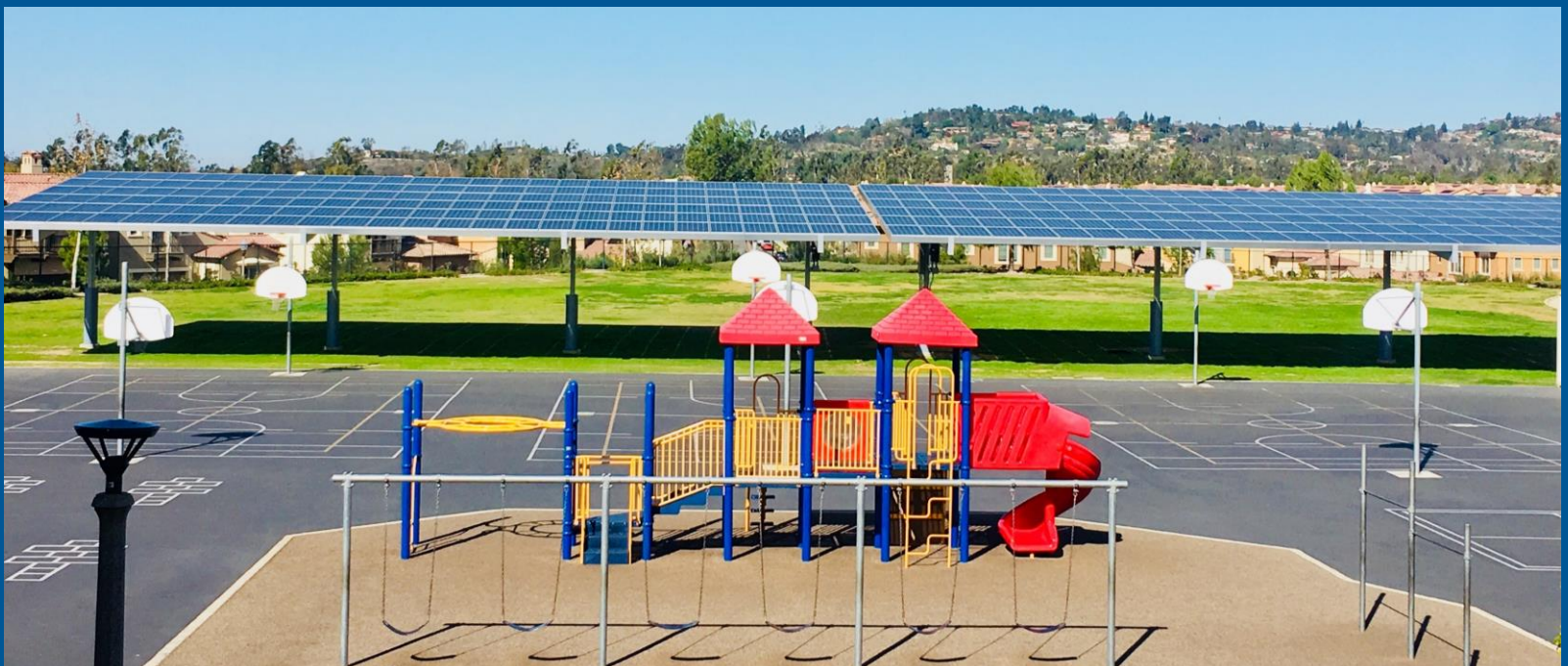
Example of an Elevated Structure
