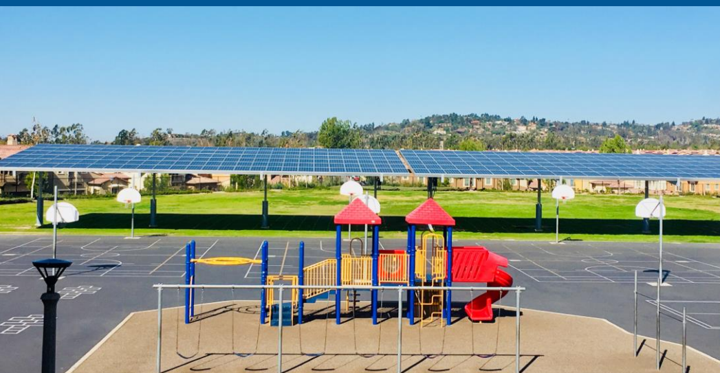
Example of an Elevated Structure
