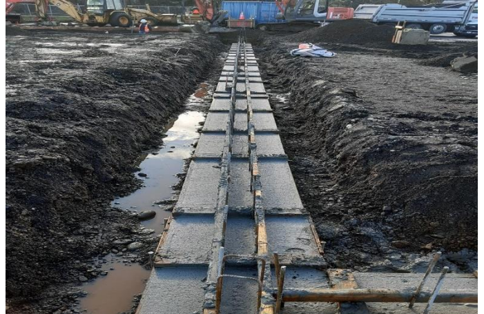
Footing concrete was poured on November 19.
