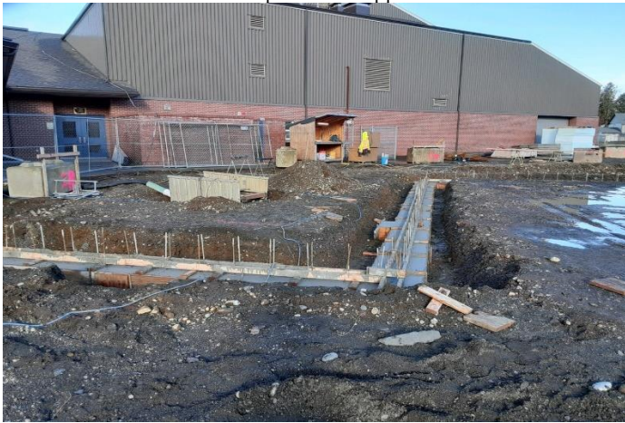
Footing forms will now be stripped.
