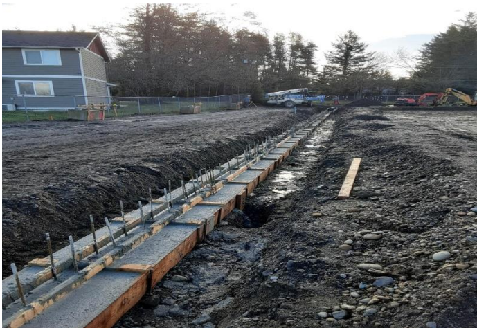
The east side forms for the classroom addition.
