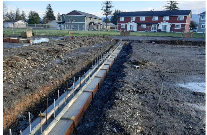
Next step will be forming the concrete stem walls.
