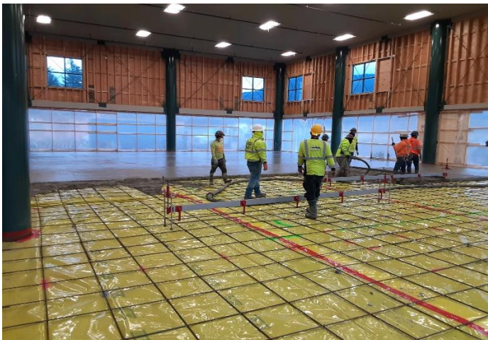
Concrete placement in action.
