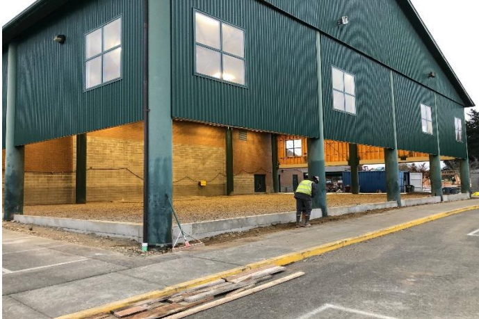
Perimeter compaction for the new exterior drains lines is nearing completion.
