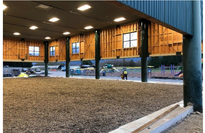
The capillary break gravel has been placed in the new gym.
