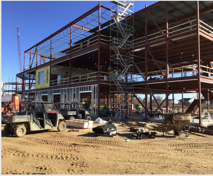
Steel Studs have started to go up at the Learning Communities
