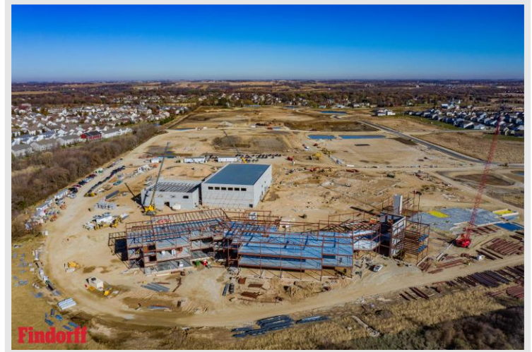
An aerial photo showing the overall progression of the building
