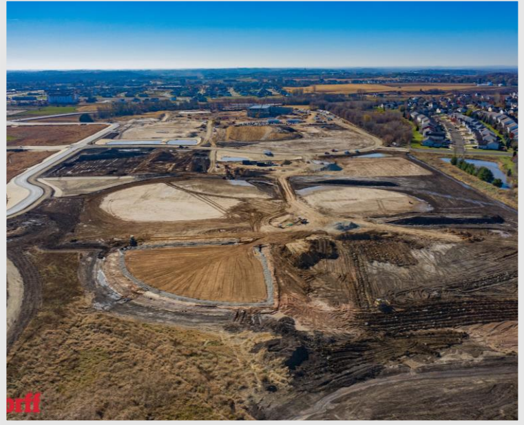
An aerial photo showing the earthwork progress on the Sports fields on the North end of the site
