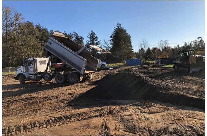
Structural fill material being delivered.
