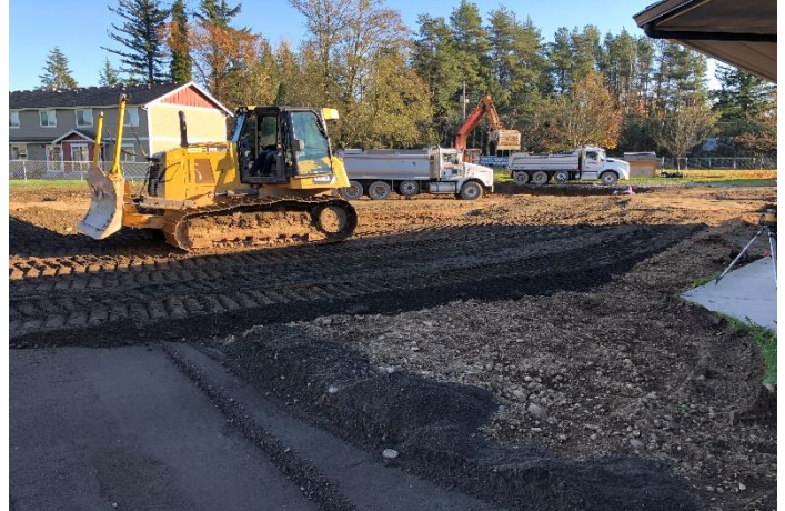
Fill material is being spread in place.
