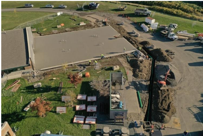
Concrete finishers just wrapping up.
