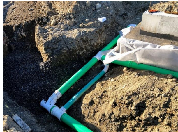
Drainage pipe installation underway.
