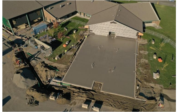
Freshly poured concrete slab.
