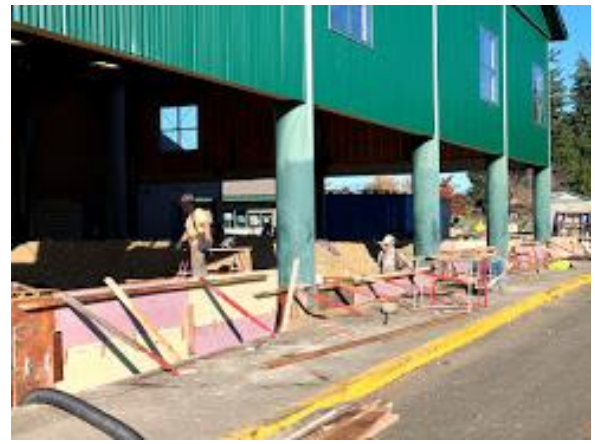
Concrete wall forms going in at play shed.
