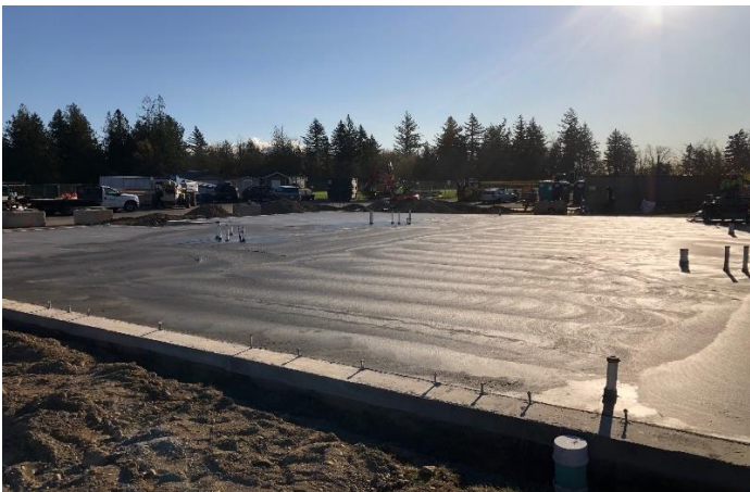
Waiting for concrete to cure enough to start finish troweling.
