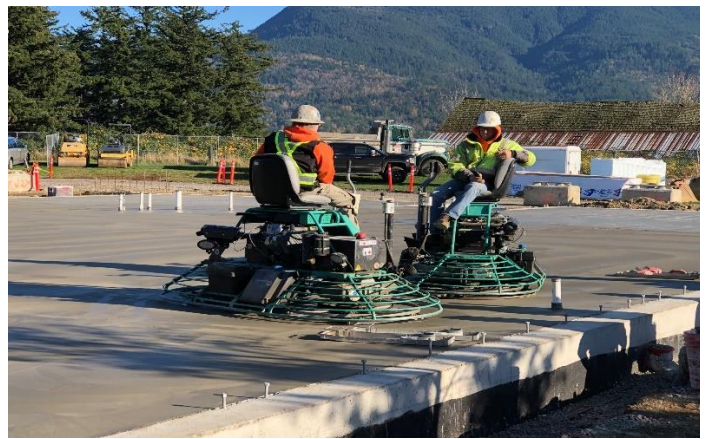
Riding power trowels preparing to start finishing the slab.
