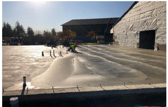
Hand trowel work underway.
