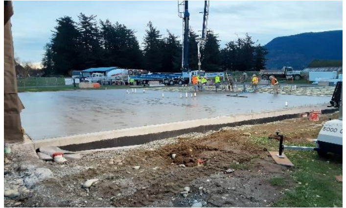
7:00 a.m.: Pump truck and concrete crew working away.
