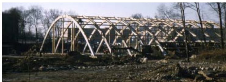
Alumni Hall, a 2,479 seat multi-purpose facility on the campus of Fairfield University and Fairfield Prep, opened on Dec. 5, 1959, and became well-known for its raucous atmosphere. It's one of the earliest pre-stressed concrete structures of its kind ever attempted. Engineering magazines from the time noted that the eleven 160-foot pre-cast arches used in the building's construction were a record-breaking span for pre-cast arch ribs used in the United States.
