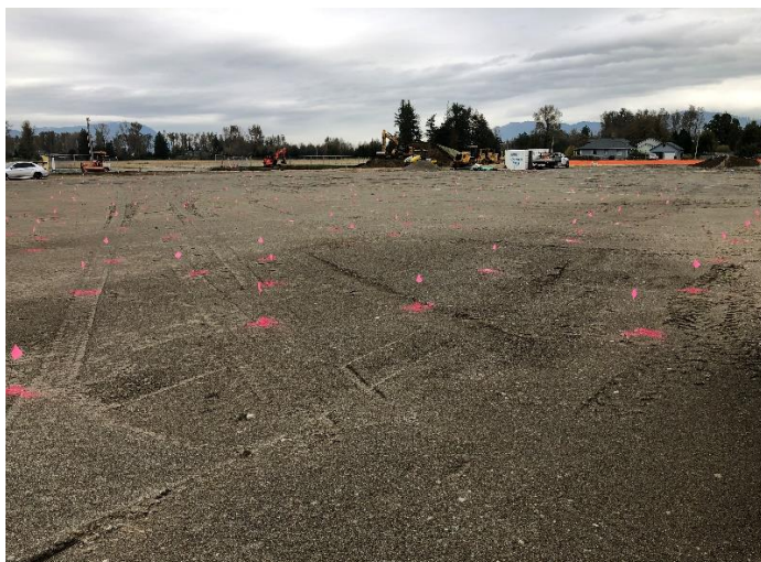
Another view of the compacted building pad looking toward the northeast.
