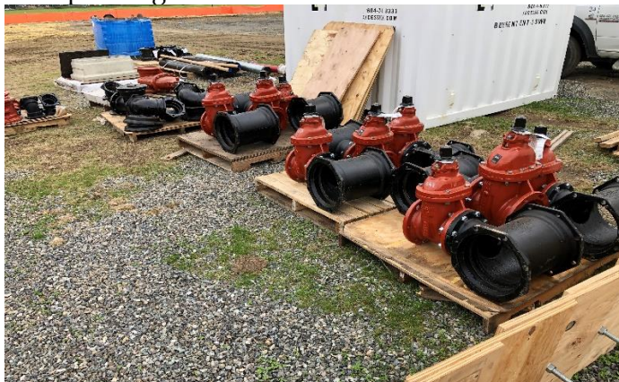
Fittings for the new upgraded water line and fire hydrant line have arrived.
