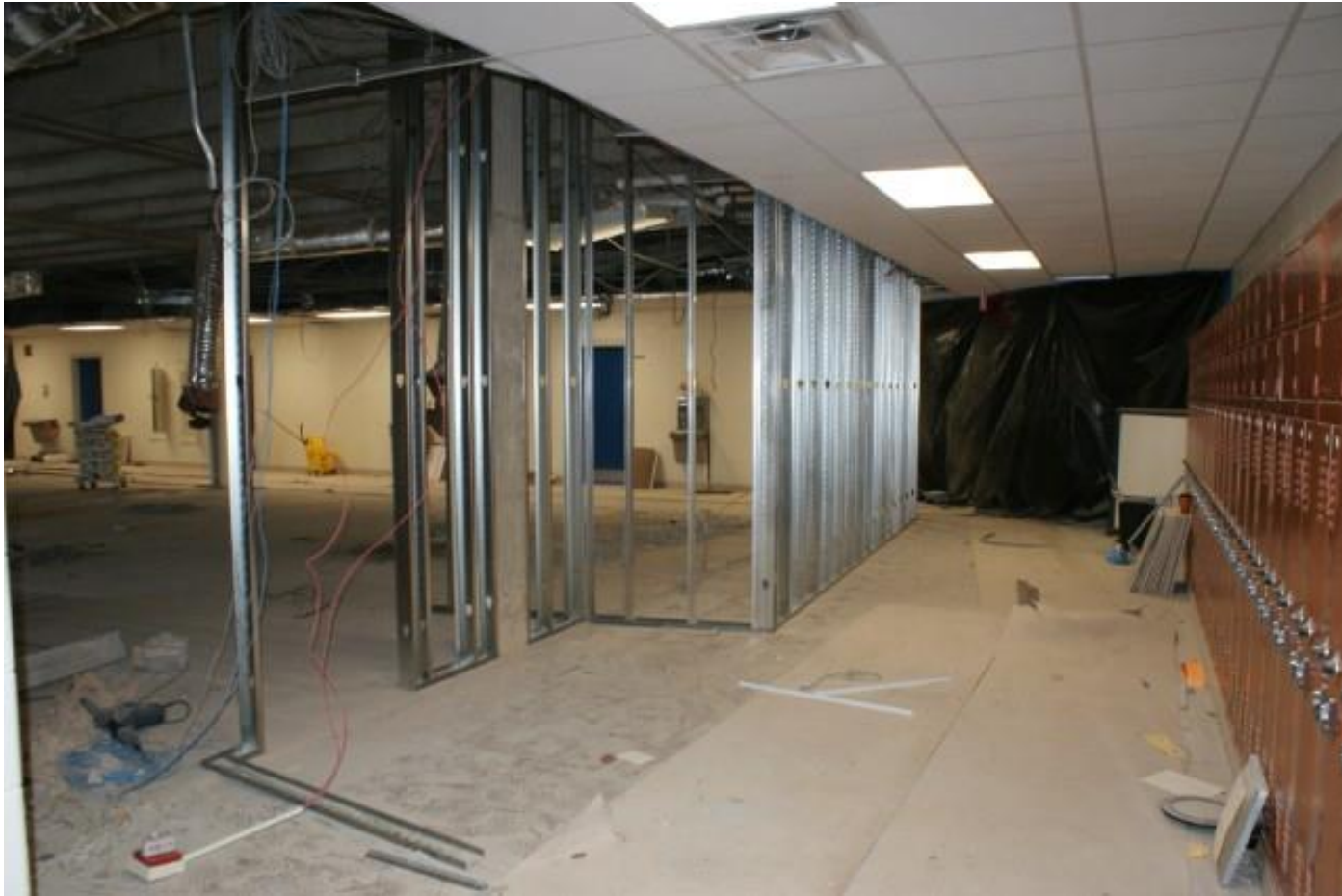
WAHS Classroom Modernization underway
