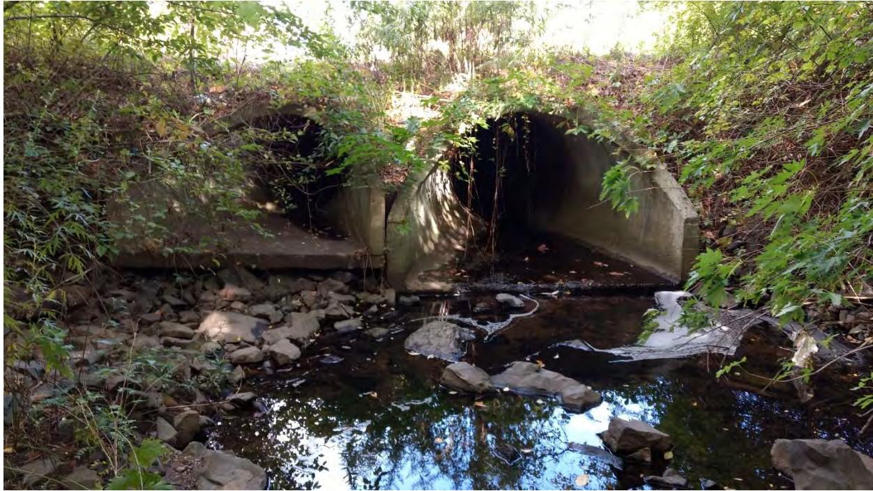
**Junction Chamber at Manhole 2 near Lindy Lane, with Debris inside Chamber**
