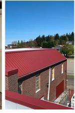
At Old Redmond Schoolhouse, the new roof is complete. Construction crews are also finishing restoration of windows and masonry. Installation of new siding is nearly complete. Inside, painting is complete. Work continues on other aspects of construction, including floors, ceilings and casework. The renovated building is scheduled to open with 10 preschool classrooms this fall.
