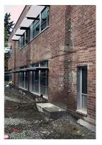
Exterior brick veneer is complete and painting is about halfway complete inside the Lake Washington High School classroom addition. Crews completed installation of the exterior glass window panels this spring as well as the elevator. The 20-classroom addition is scheduled to open this fall.
