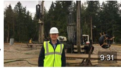
Drilling of geothermal heating at new middle school in Redmond...
