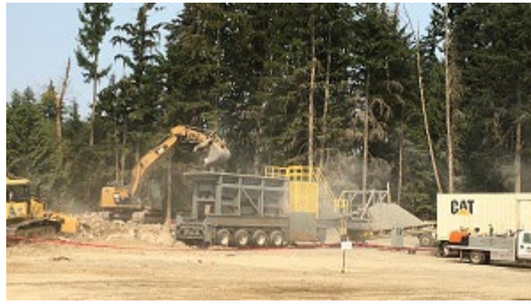
Photo: Rock crushing at the New Middle School in Redmond Ridge.
