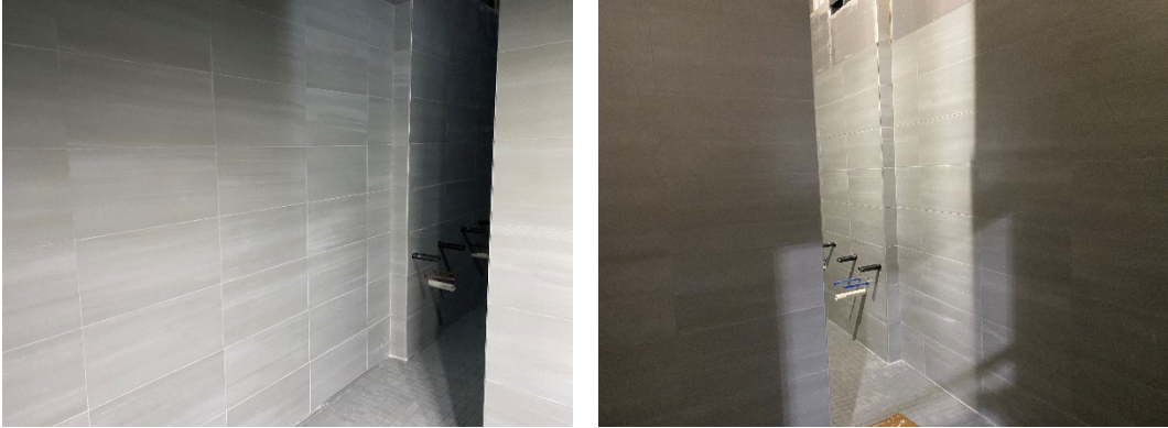
Middle School – Area D Bathroom Tile Installation
