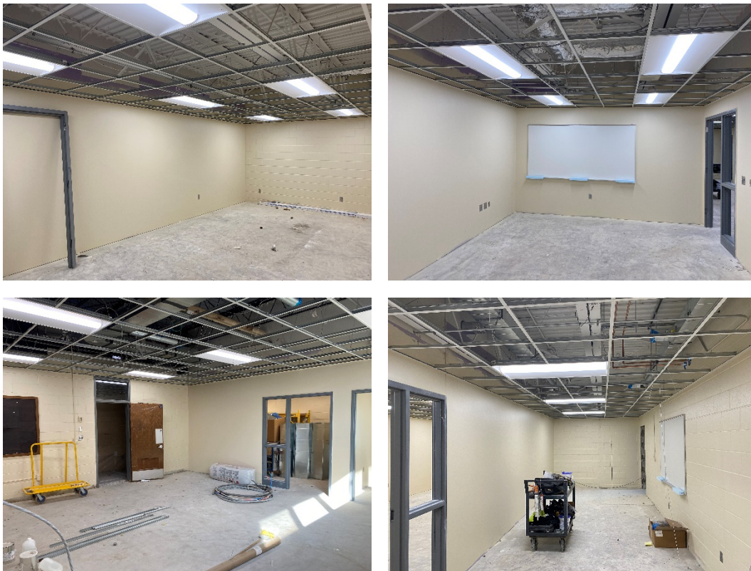
Middle School – Area D SPED Classroom Ceiling and Lighting Installation
