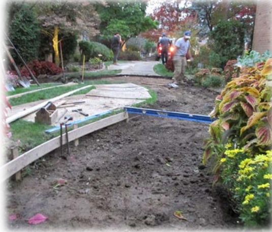
The removal of the old cement.
