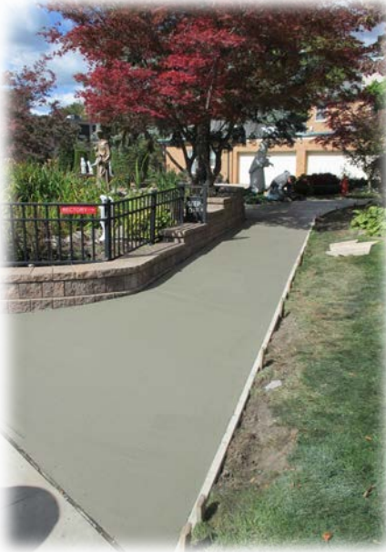
Freshly poured concrete.
