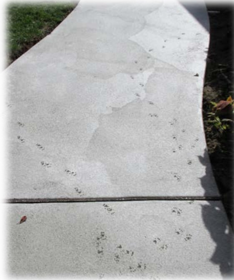
A little critter decided to walk across the newly poured concrete. Thankfully, it was fixable!
