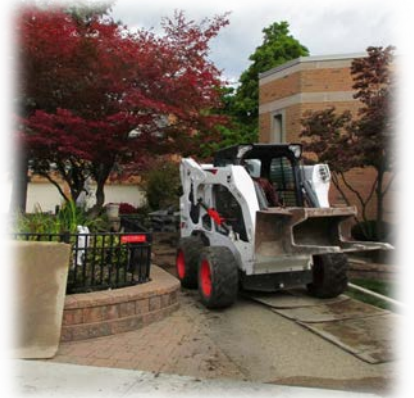
The Rectory walkway gets a new concrete path!
