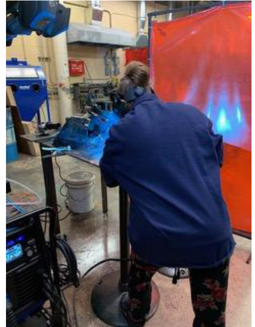
East High School student Lindsey Lawton welds a lap joint in the welding lab at school. She plans to intern at a local business after graduation in preparation for a career in welding.
