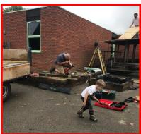
Installing a waterproof roof on the shelter near the infant's door and strengthening the uprights to ensure it remained solid. The shelter is used for breaktimes, reading sessions and FoBIPS bake sales so it is crucial to protect occupants from the elements.
