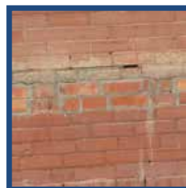
Failing masonry
