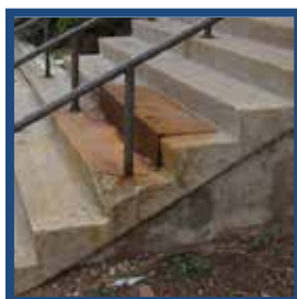
Failing concrete
