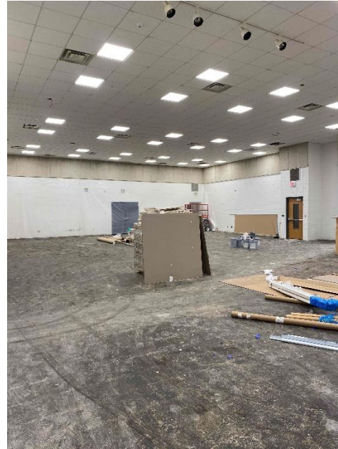
CCES – Cafeteria/multi-purpose ceiling complete
