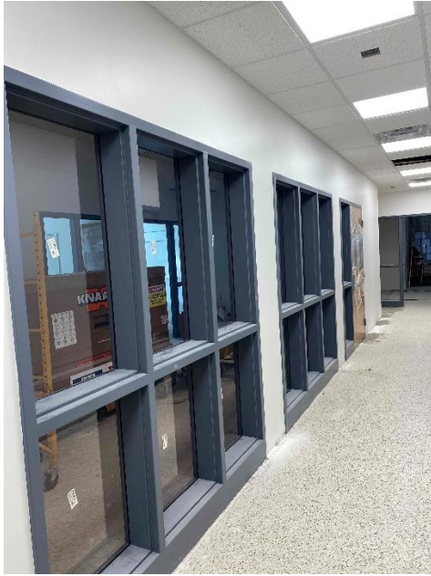
CCES – Glass, flooring, and ceiling complete in area D SPED suite
