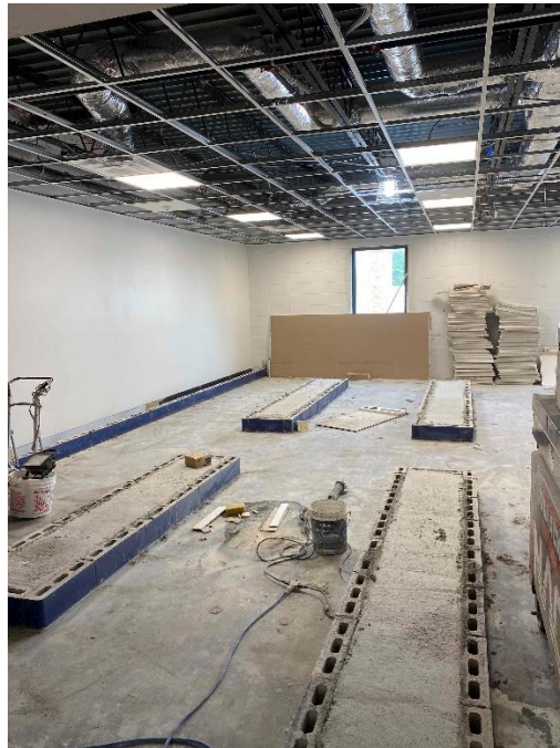
SFMS – Locker bases installed in upper C/D locker commons
