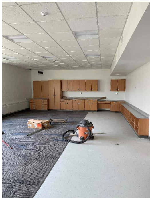
ECFC – Casework installed in area A classrooms
