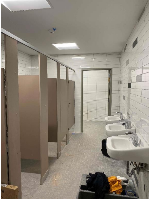
SFMS – Lower C bathroom plumbing fixtures and partitions are installed
