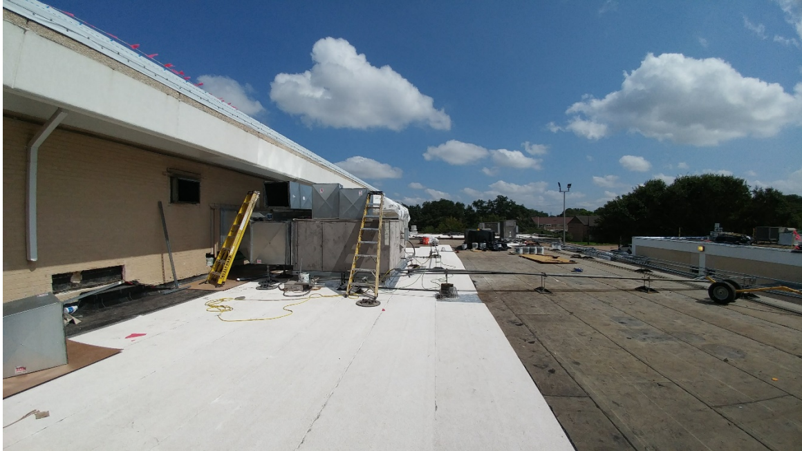
Roof Cap sheet installation in progress at Area A East side.
