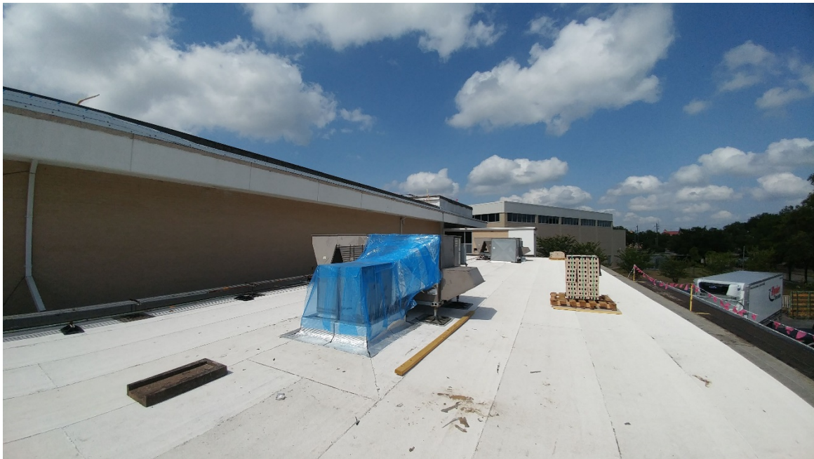
New Mechanical roof curbs and roof ap sheet Installed at Area A North side.
