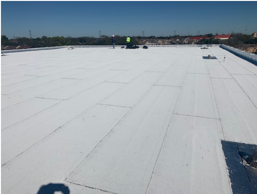
Roof Area D
