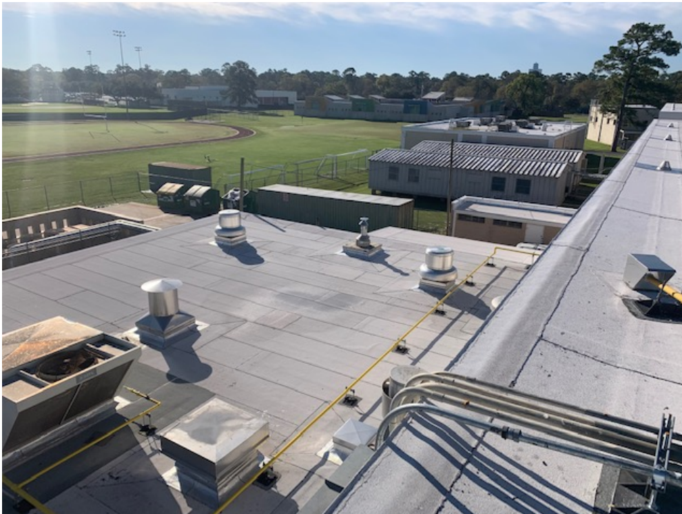
View toward roof area F.
